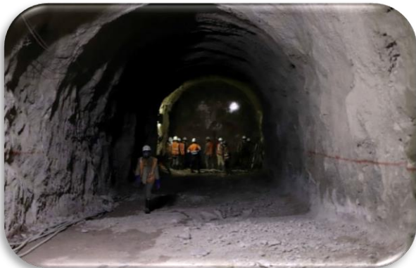
Main Decline Ramp in Construction
